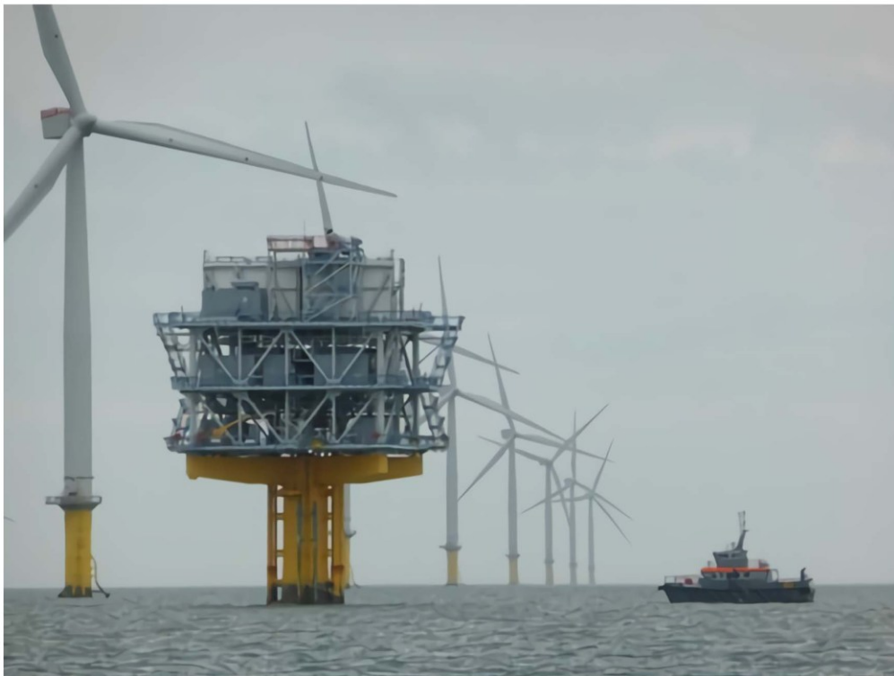
Figure 3.6 Example of an offshore substation
